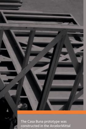
The Casa Buna prototype was constructed in the Arcelor Mittal facility in Pantelimon, Bucharest. It uses a steel frame superstructure, steel roof tile system, steel rainwater extraction system and a steel cladding. The model has been tested for energy efficiency and carefully assessed to ensure comfort and adequate living space.
