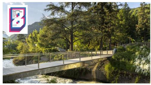
The girders of the Brides les Bains footbridge are made of Aperam 304L stainless steel, with a Uginox polished mirror reflecting the eddies and movements of the water. The footbridge thus changes with the seasons and the weather, and allows for discrete integration into this alpine environment.
