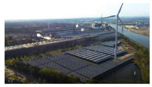
> The 50,000 panels installed in Genk (left) started providing green electricity to the site at the beginning of 2022. Almost 20 GWh were produced during the year, covering nearly 5% of the site's electricity needs. We are investigating how to increase this capacity. We are also installing LED lighting, which helps save an additional 6000 MWh annually.
