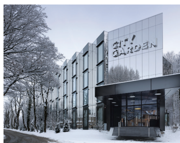
Hotel City Garden, Zoug - Switzerland EM2N Architekten AG Ghisleni Planen Bauen Gmbh MZ-IMMOBILIEN AG. Executed using grade 304 / 1.4301 with Uginox Méca 8ND finish © Aperam
