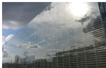
Archives Départementales du Bas-Rhin, Strasbourg. Architect: Bernard Ropa & TOA Double skin glass / stainless steel Executed using grades 304 / 1.4301 with Uginox Méca 8 ND finish © Bernard Ropa
