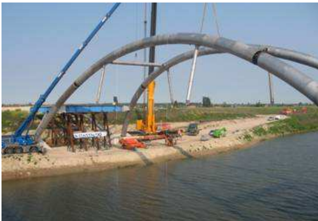
Bridge arches in construction in 2304
