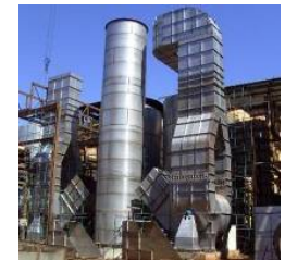
Carbon steel substitution
