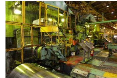
Timoteo - Sendzimir Mill #1 upgrade
